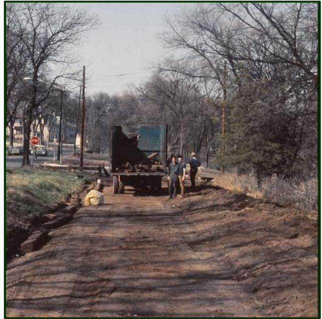
(Above and Above Left) Ya gotta start someplace, eh? Here are two 1970 photos. The top left photo shows the foundation for the first single-car car barn has been finished and it looks like the crew is leveling the earth for the first set of ties to be delivered. In the above photo, ties are being delivered to the newly graded right-of-way. You can't see them very clearly, but those ties look very used. That's west 42 nd Street directly in front of the truck. (Left) First day of operations was on August 28, 1971. No. 1300 looks pretty nice making one of the runs on this momentous day. (Three photos by Bill Cordes)
